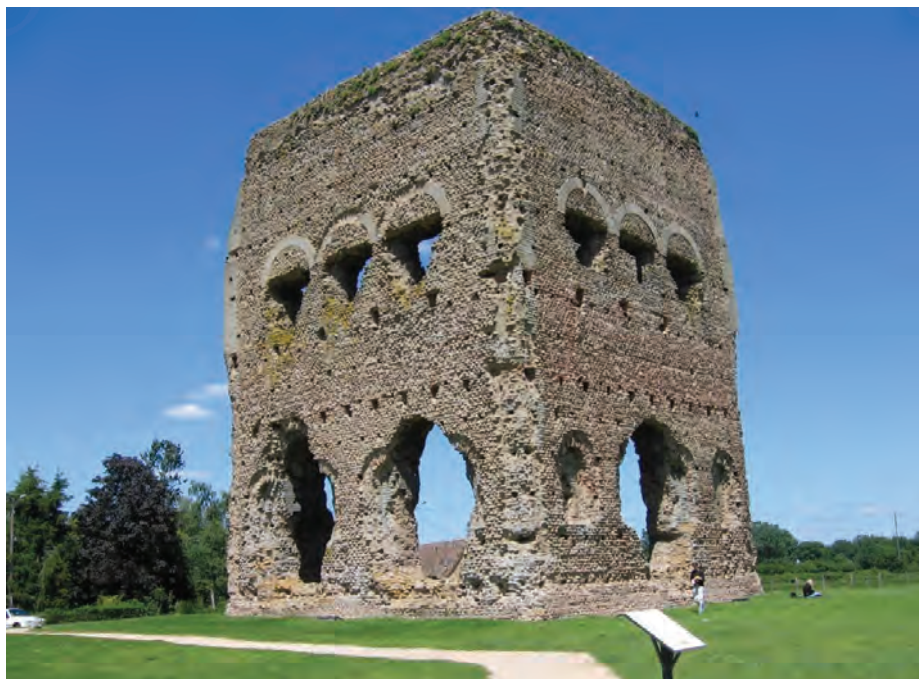
The temple of Janus (Autun) showing the surviving central cella. The slots for the beams of the surrounding ambulatory roof can clearly be seen in the masonry.
